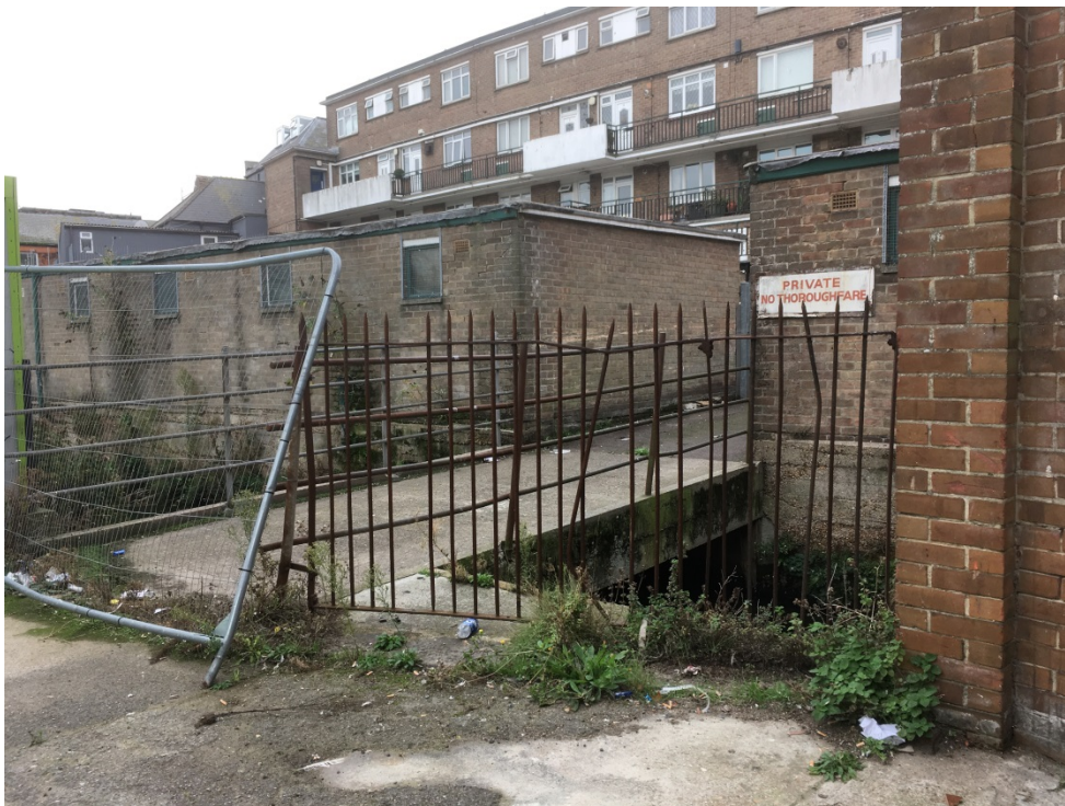
Dolphin House Rear Yard Bridge
